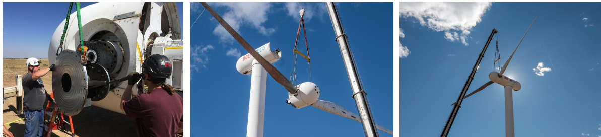
(a) NWTC technicians install one of the blade adapters to the CART2 hub.
