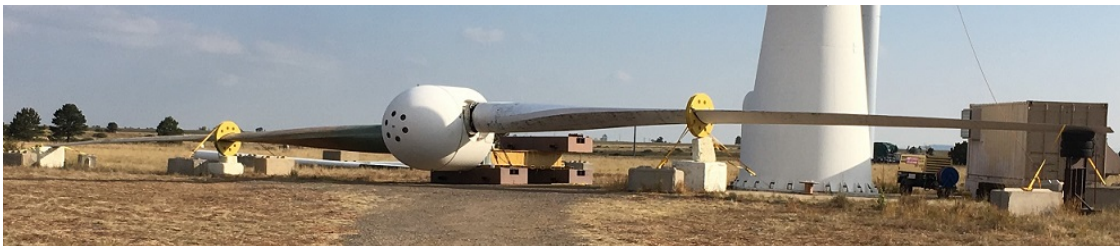
(a) Rotor-hub assembly on cradle.
