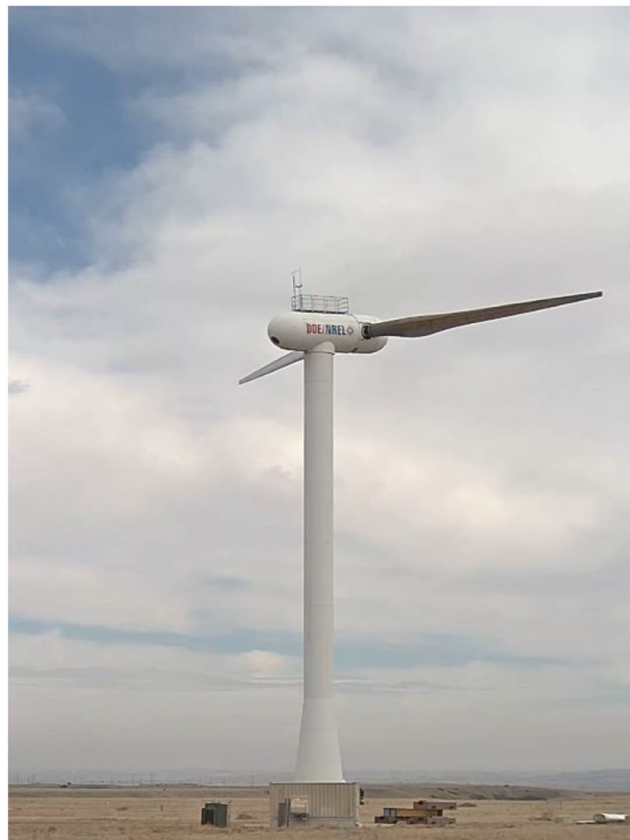
FIGURE 1 The SUMR-D blades mounted on the two-bladed CART-2 at the NREL FC and placed in parked conditions
