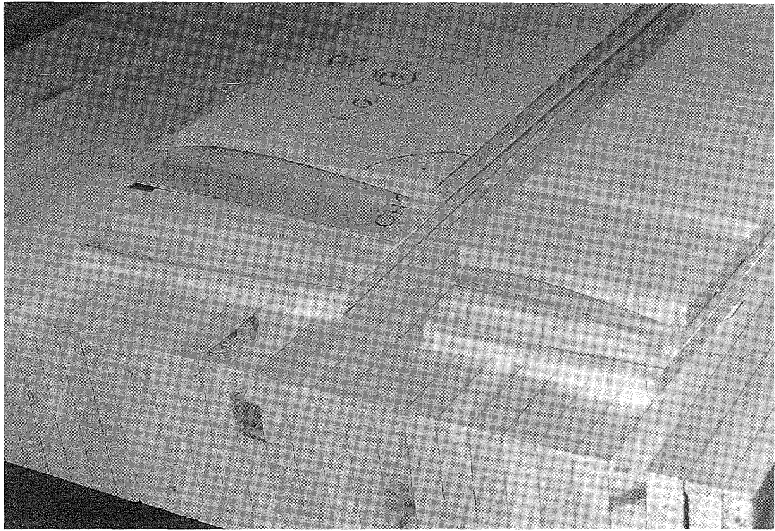
Figure 1: Blue foam cores with the prefabricated fiberglass skins. Skins will be epoxied to foam cores. They consist of a 295 grams per square meter (about 1 ounce per square foot) glass cloth soaked with epoxy resin.
